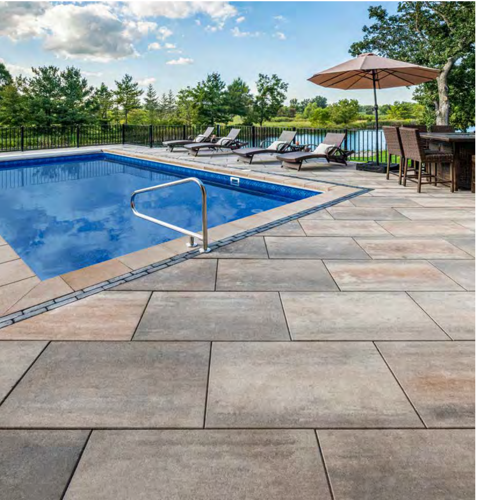
Pavers: Beacon Hill™ Smooth Slab(Bavarian Blend) with Copthorne®(Basalt) accent Retaining Wall and Grill Island: U-Cara® Smooth(Bavarian Blend)
